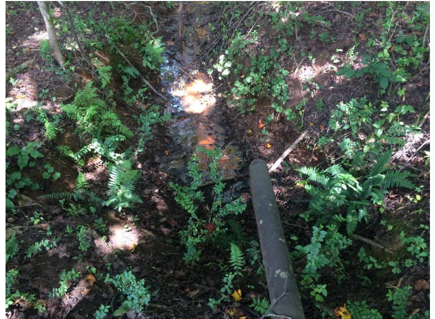
Photo 2: View of piped culvert from the pond discharging to stream S3.
