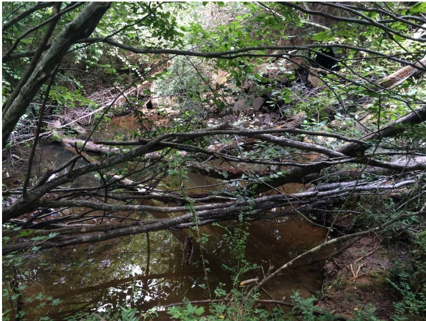
Photo 7: View of the culvert from the large pond to the east of the site discharging into Wetland A.
