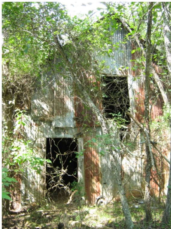
Figure 17. View of standing barn, facing west.
