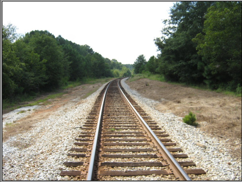
Figure 19. View of CSX/Georgia Railroad, facing west.
