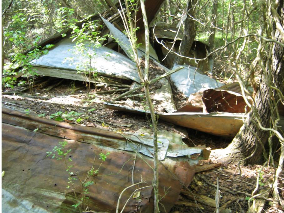
Figure 18. View of collapsed barn, facing southwest.
